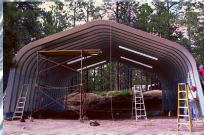
STEP 3 Raise arches into place
