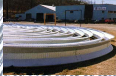
STEP 2 Bolt arches together on the ground
