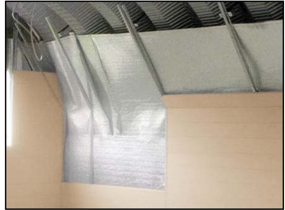
Semi-rigid Board over EZ-Roll (Mounted on furring strip)
