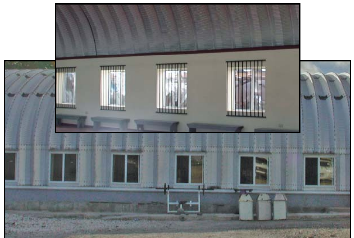
Windows in Side Panels
