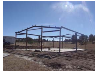
Attach wall girts and mainframes
