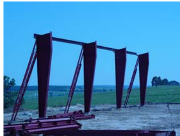
Stand main frame columns
